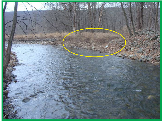
Location B. Looking downstream at new diversion point. Flow left of oval is now shunted into the Bashakill Marsh versus southwest of wetland in former channel.
