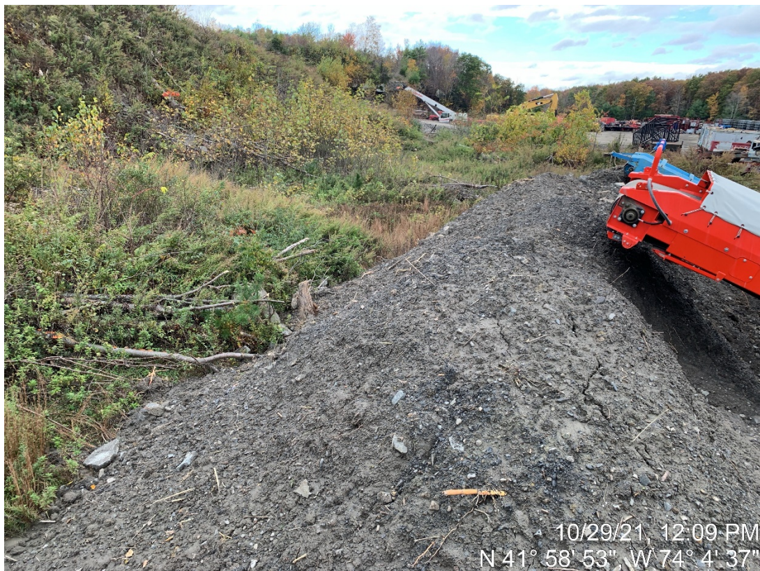
Photo 12: Material Stockpiles with no erosion controls.
