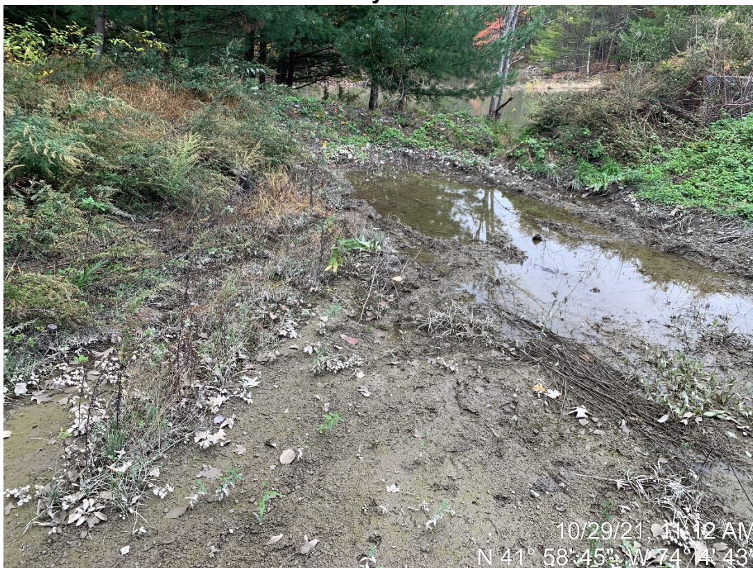
Photo 4: Cut in berm to Pond D with signs of turbid discharge.
